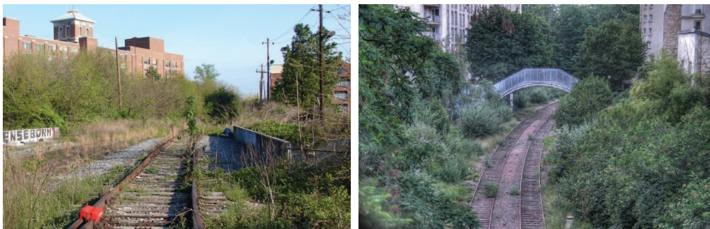
Abandoned infrastructure at the Atlanta BeltLine (left) and the Petite Ceinture in Paris (right)
